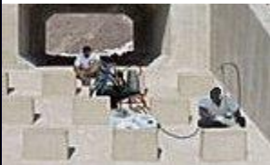
(Above) Completed spillway
